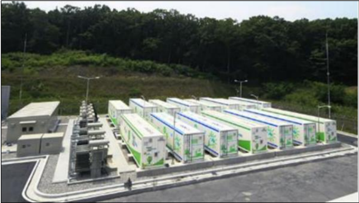
Figure 8: Example of a 15-container Lithium-Ion BESS installation.
